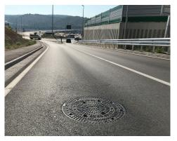
ACO provided HSD-2 bridge drains for its closed drainage system together with CityTop P Bituplan manhole covers, also build on access roads towards the bridge.
