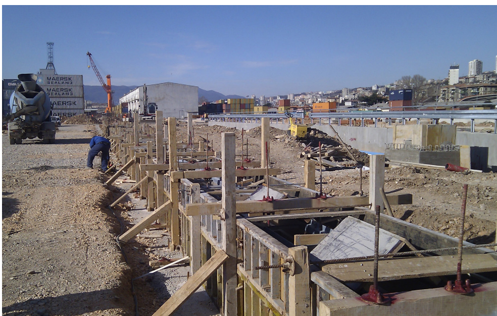
Construction site at the time of installing of ACO Aquaduct channels
